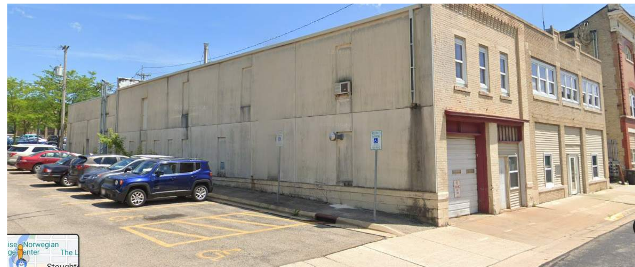
EXISTING NORTHWEST FACADE
