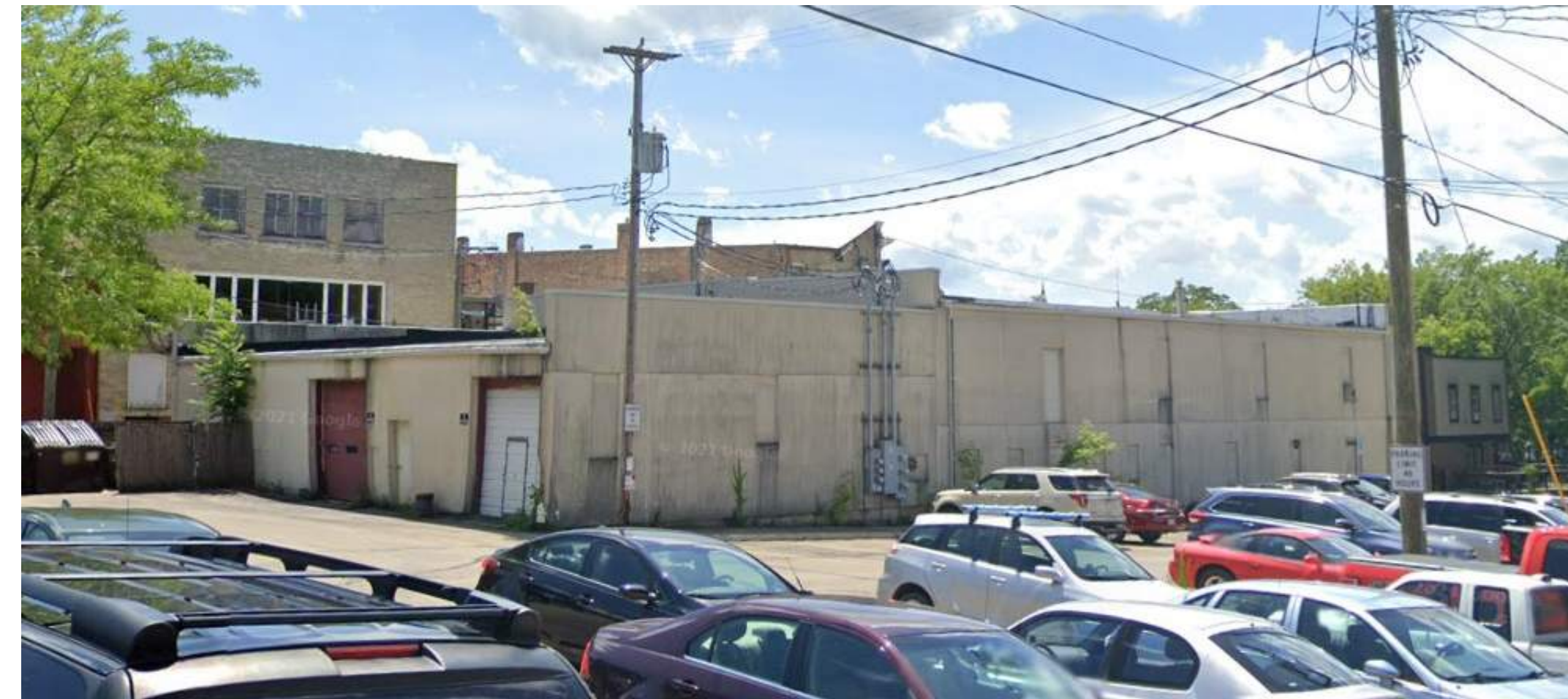
EXISTING NORTHEAST FACADE
