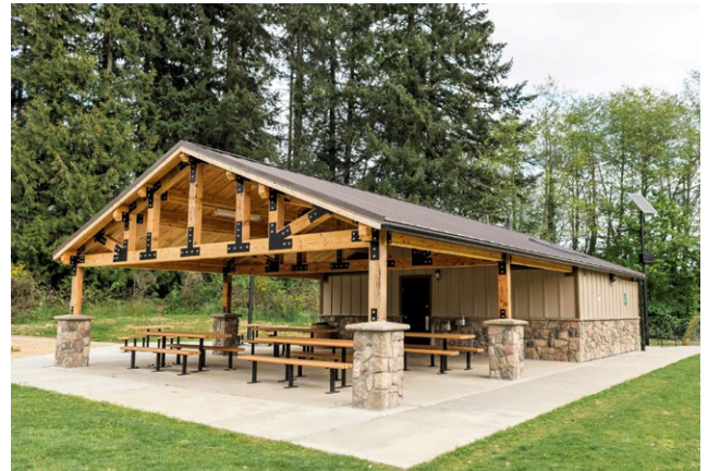
Figure 4.1: Example Shelter and Restrooms
