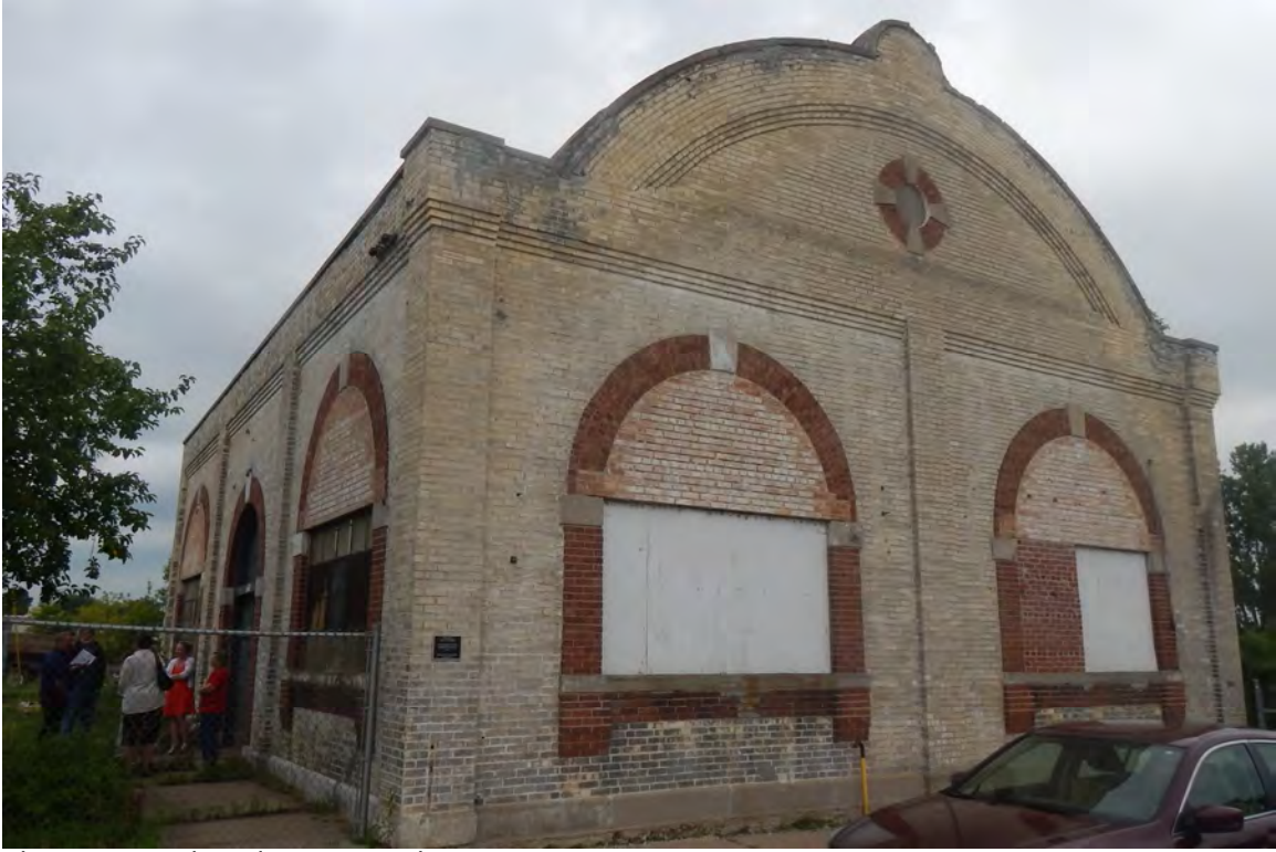
Photo 2 - North and West Facades
