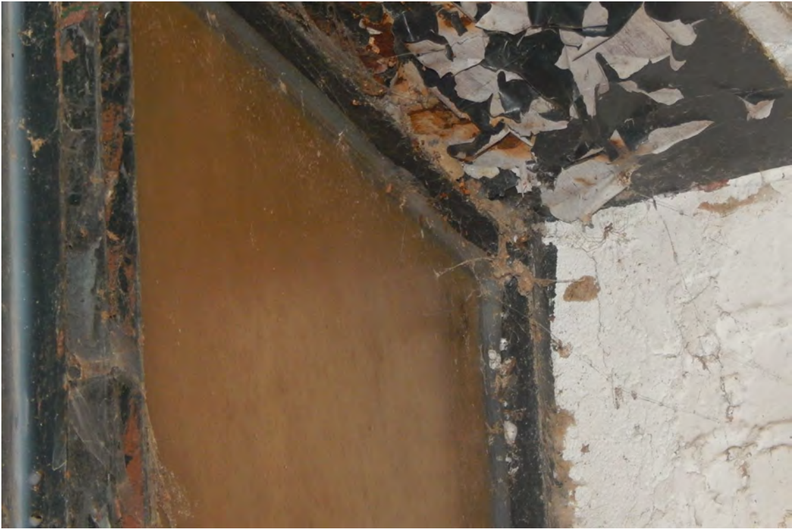
Photo 15 - View of original steel sash window
