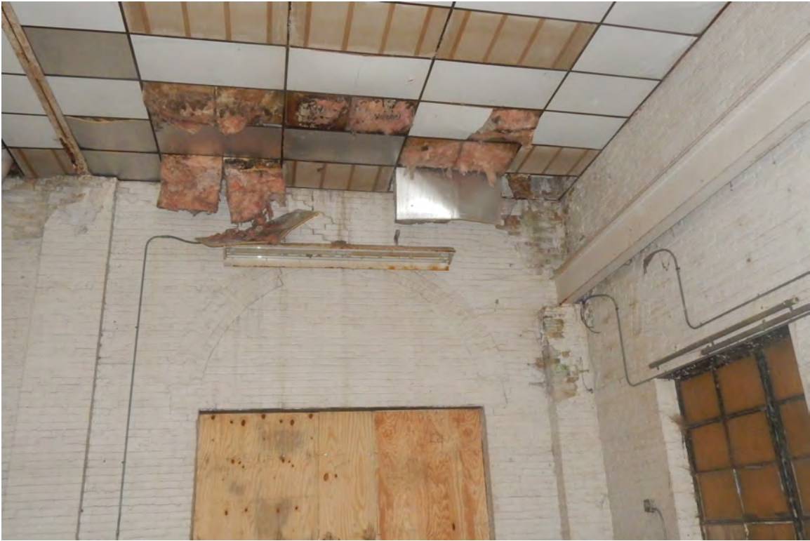
Photo 12 - View of interior condition (lay-in ceiling and existing steel sash windows)
