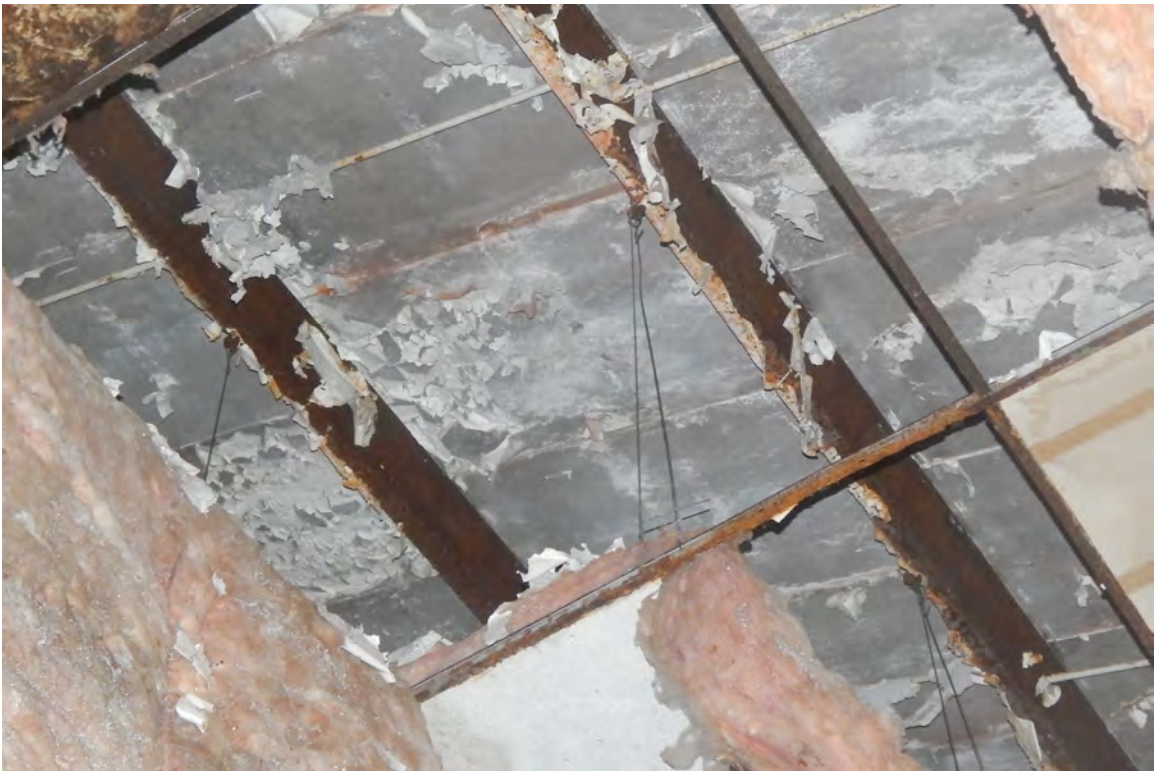
Photo 16 - View of precast concrete infill panel
