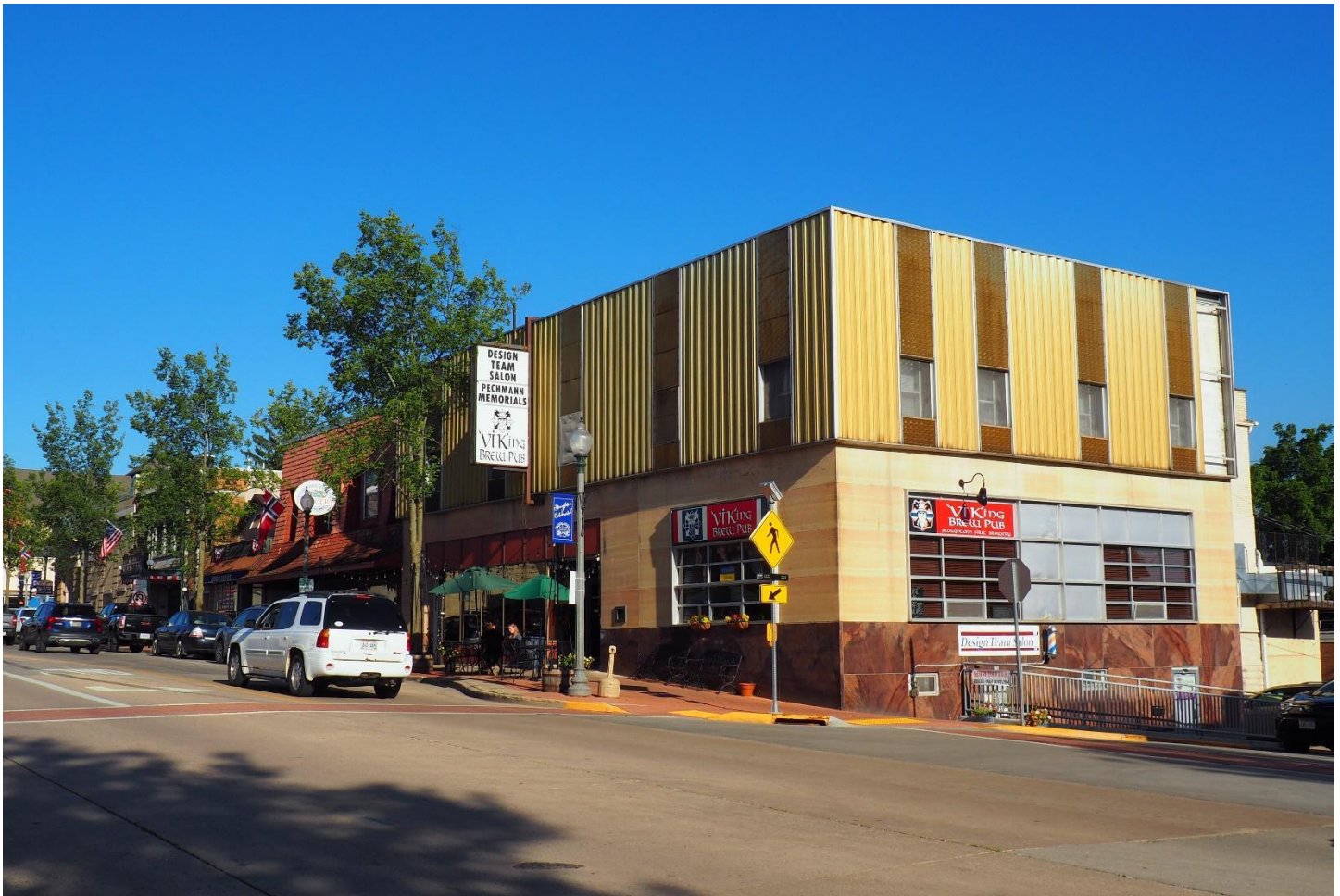
PHOTOGRAPH 14 OF 22: VIEW OF THE WEST HALF OF THE SOUTH SIDE OF THE 200-BLOCK OF E. MAIN STREET LOOKING SOUTHEAST.
