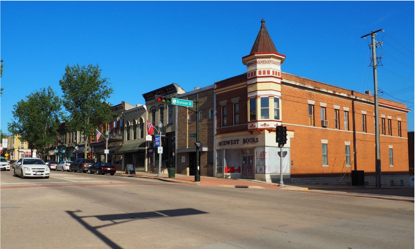
PHOTOGRAPH 10 OF 22: VIEW OF THE WEST HALF OF THE SOUTH SIDE OF THE 100-BLOCK OF E. MAIN STREET LOOKING SOUTHEAST.
