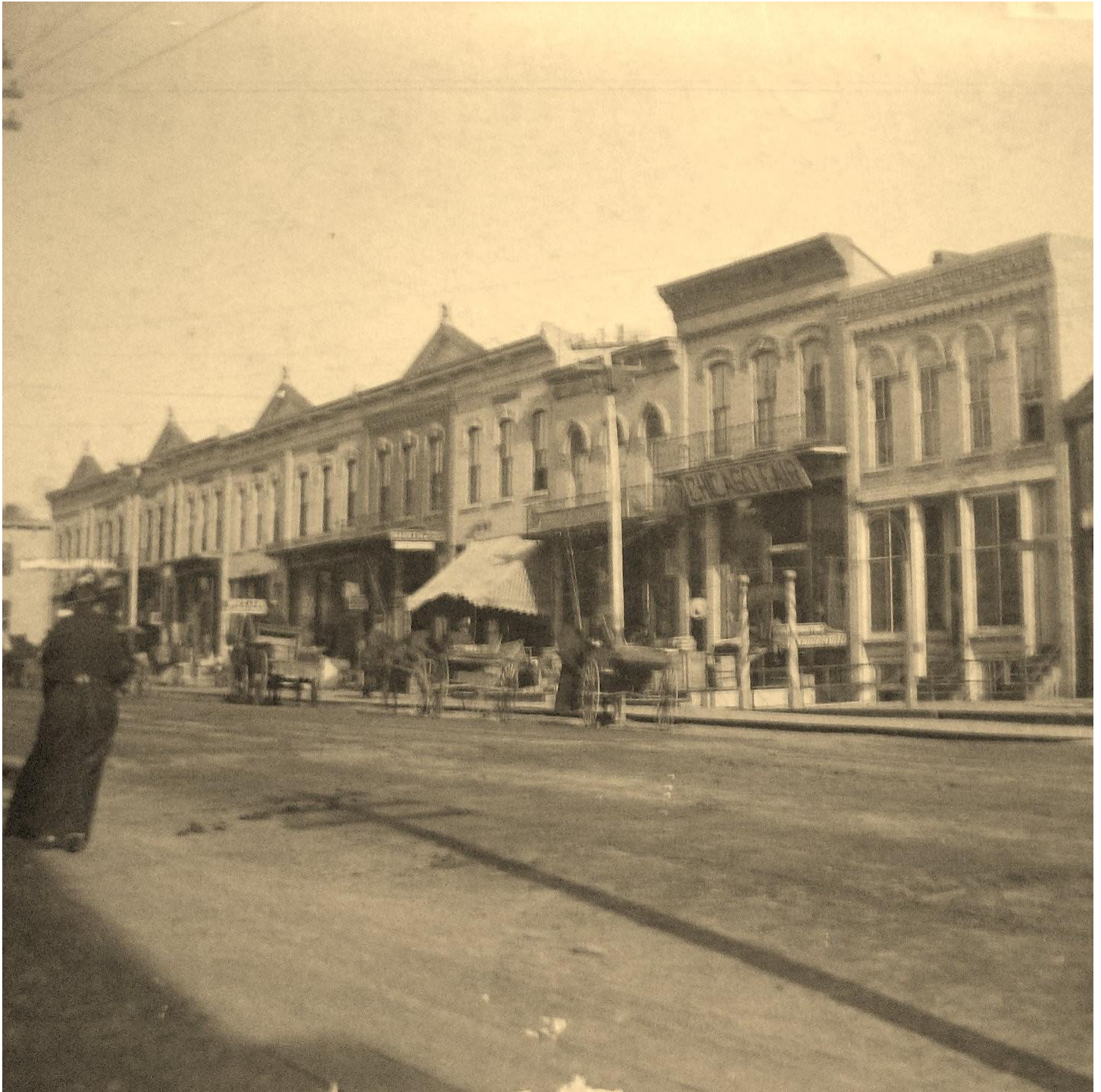
HISTORIC PHOTOGRAPH 1 OF 21: VIEW OF THE SOUTH SIDE OF THE 100-BLOCK OF E. MAIN STREET, UNDATED. COURTESY OF THE STOUGHTON HISTORICAL SOCIETY.
