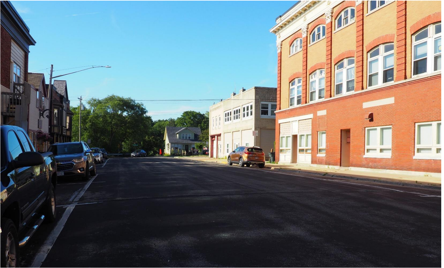
PHOTOGRAPH 3 OF 22: VIEW OF THE 200-BLOCK OF S. WATER STREET LOOKING NORTH.
