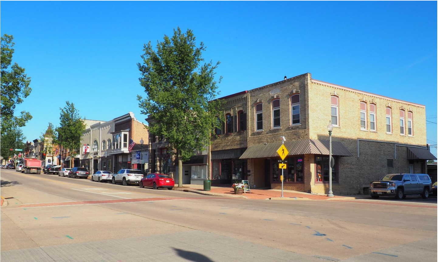
PHOTOGRAPH 4 OF 22: VIEW OF THE SOUTH SIDE OF THE 100-BLOCK OF W. MAIN STREET LOOKING SOUTHEAST.
