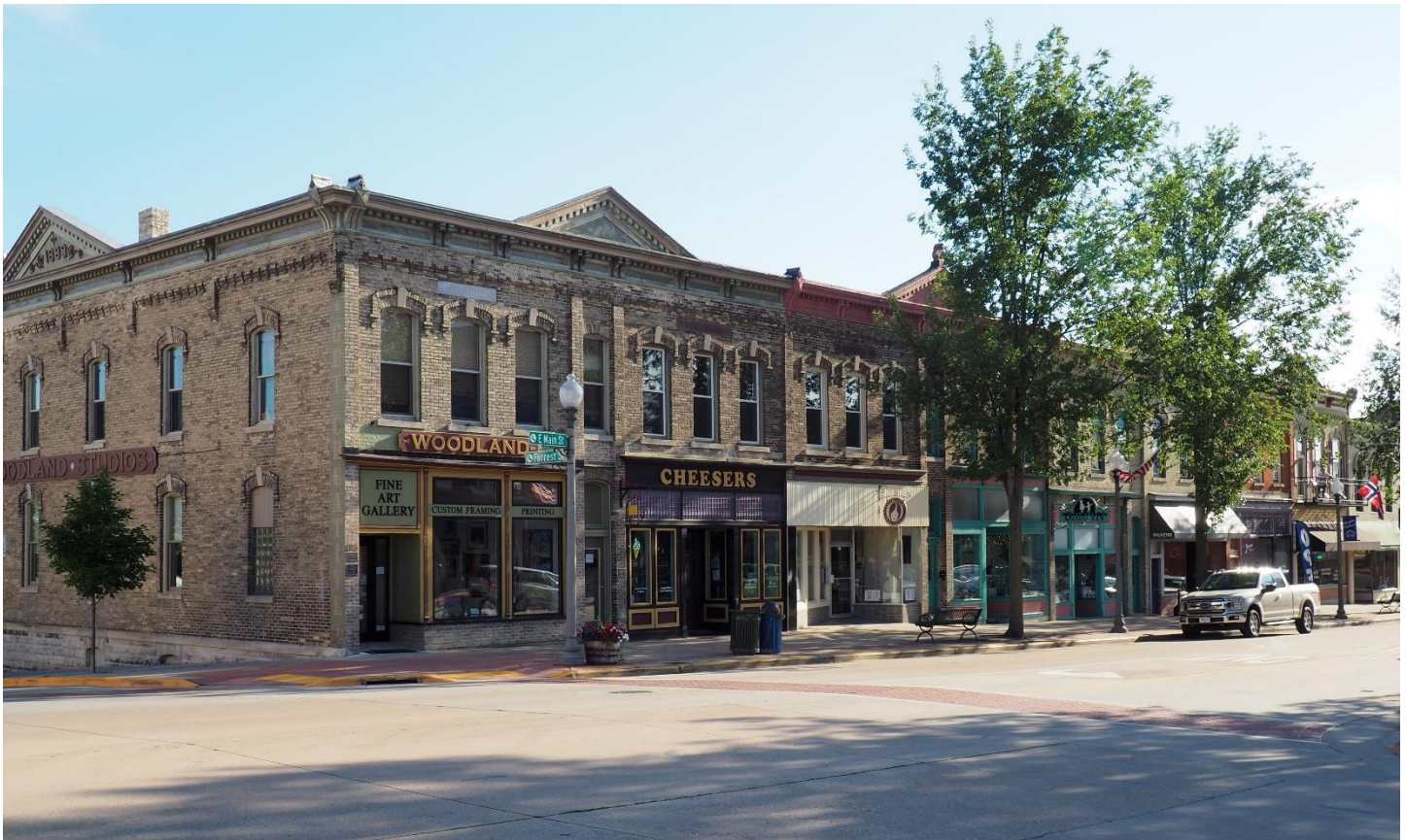
PHOTOGRAPH 13 OF 22: VIEW OF THE EAST HALF OF THE SOUTH SIDE OF THE 100-BLOCK OF E. MAIN STREET LOOKING SOUTHWEST.
