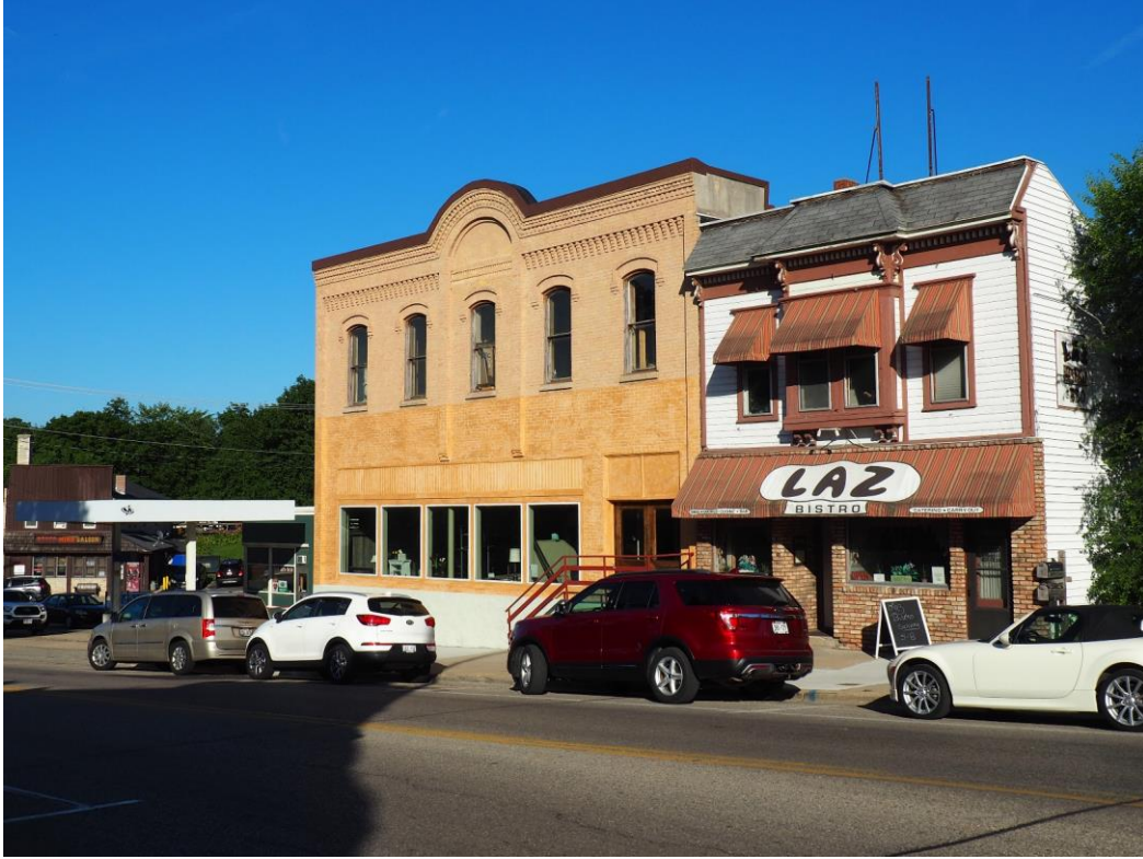
PHOTOGRAPH 20 OF 22: VIEW OF THE SOUTH SIDE OF THE 400-BLOCK OF E. MAIN STREET LOOKING SOUTHEAST.
