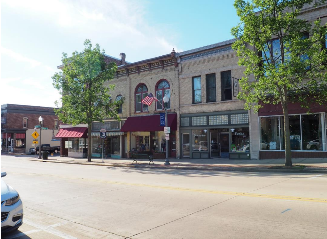
PHOTOGRAPH 6 OF 22: VIEW OF THE WEST HALF OF THE NORTH SIDE OF THE 100-BLOCK OF W. MAIN STREET LOOKING NORTHWEST.
