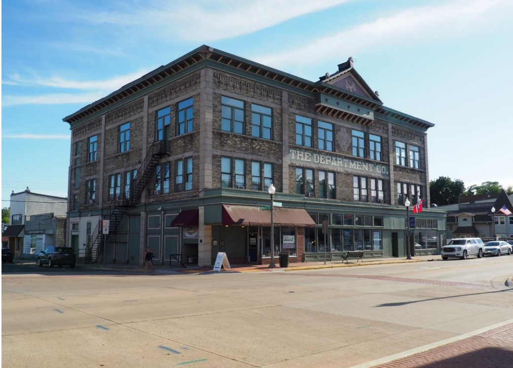
PHOTOGRAPH 1 OF 22: VIEW OF THE SOUTH SIDE OF THE 200-BLOCK OF W. MAIN STREET LOOKING SOUTHWEST.
