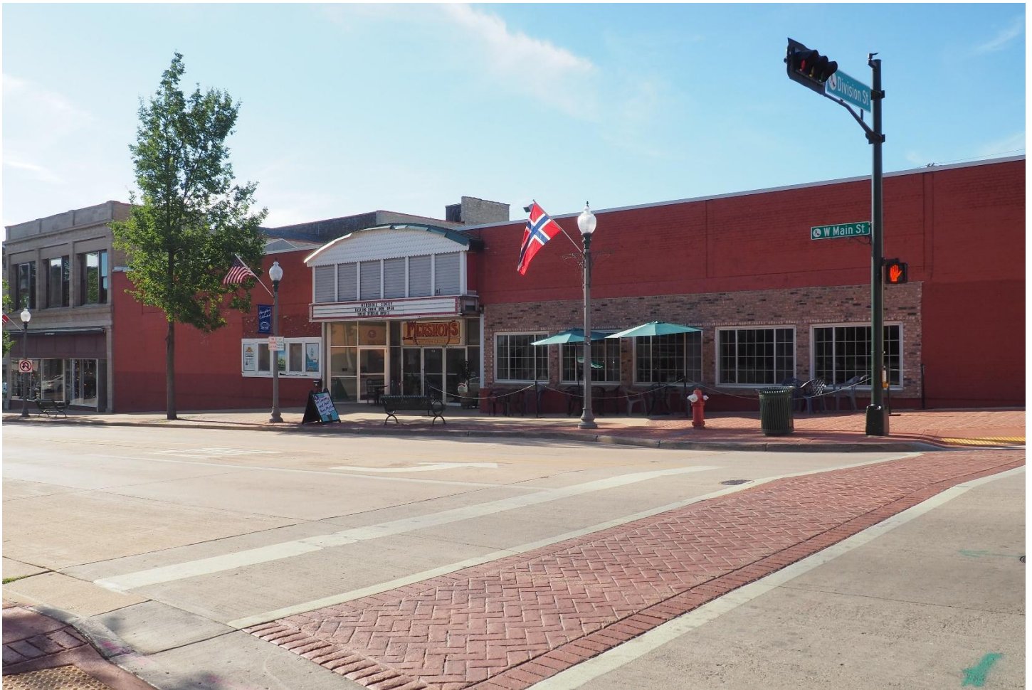
PHOTOGRAPH 8 OF 22: VIEW OF THE EAST HALF OF THE NORTH SIDE OF THE 100-BLOCK OF W. MAIN STREET LOOKING NORTHWEST.
