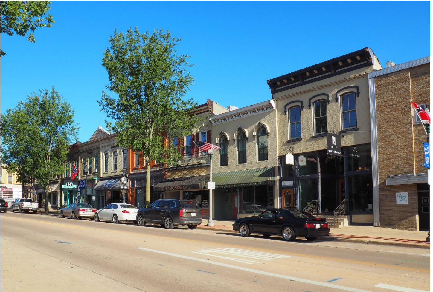
PHOTOGRAPH 11 OF 22: VIEW OF THE SOUTH SIDE OF THE 100-BLOCK OF E. MAIN STREET LOOKING SOUTHEAST.
