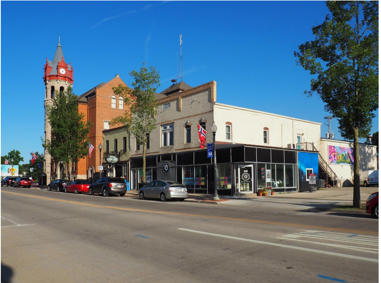
PHOTOGRAPH 17 OF 22: VIEW OF THE SOUTH SIDE OF THE 300-BLOCK OF E. MAIN STREET LOOKING SOUTHEAST.
