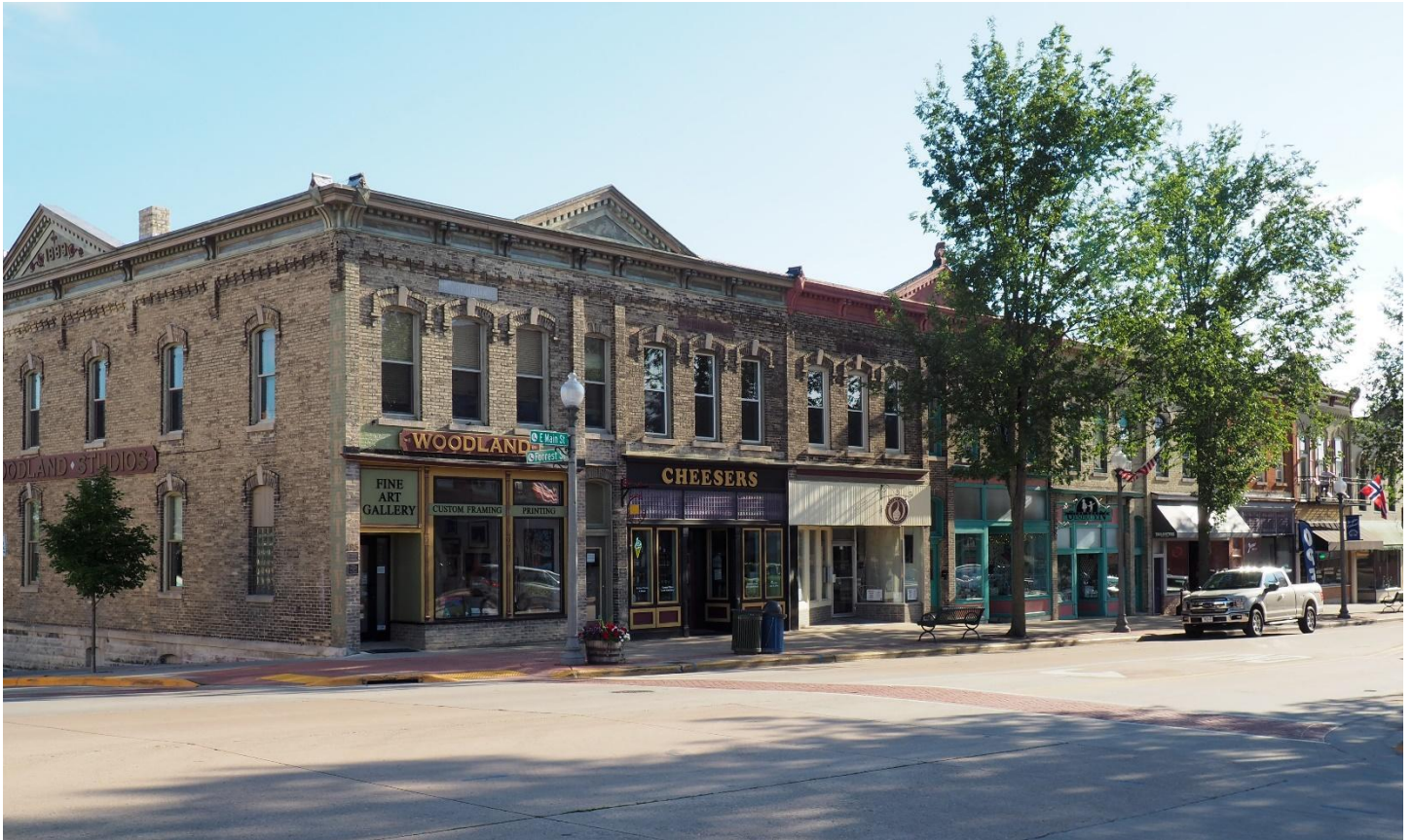
PHOTOGRAPH 13 OF 22: VIEW OF THE EAST HALF OF THE SOUTH SIDE OF THE 100-BLOCK OF E. MAIN STREET LOOKING SOUTHWEST.
