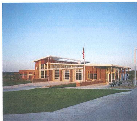
Madison Fire Station No. 12
