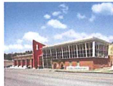
Waukesha Fire Station
