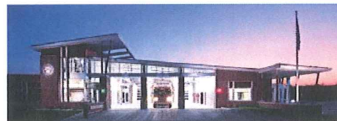
Madison Fire Station No. 12
