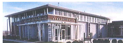
Madison Fire Station No. 11
