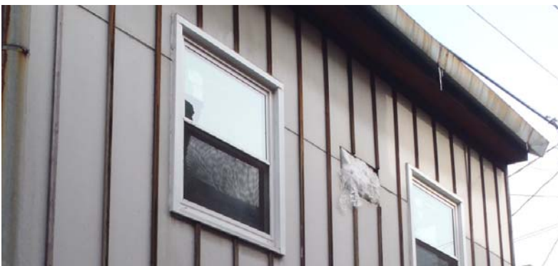
Parcel #62: Metal panel façade with insulation-filled hole (top).
