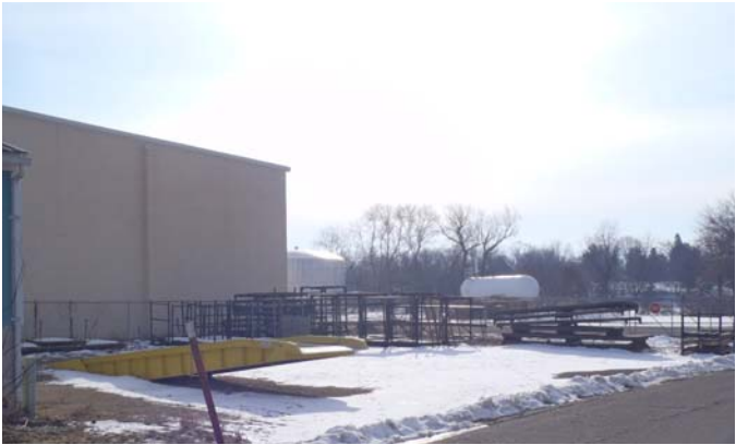
Parcel #44: Unscreened outdoor storage of items.
