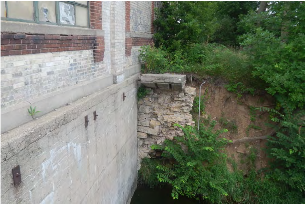
Photo 18 - View of damaged retaining wall and unstable bank/erosion
