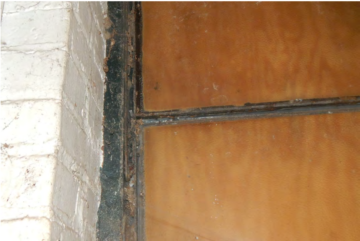
Photo 14 - View of original steel sash window
