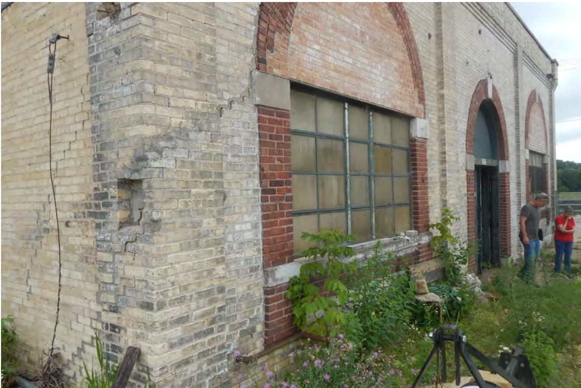
Photo 10 - Southeast Corner - Note Wall Movement
