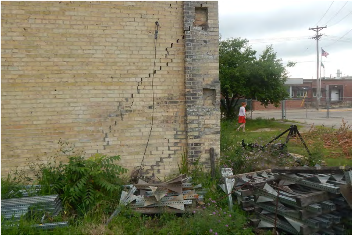
Photo 9 - Southeast Corner - Note Wall Movement
