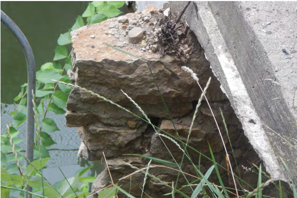
Photo 6 - Deteriorated Foundation/Retaining Wall
