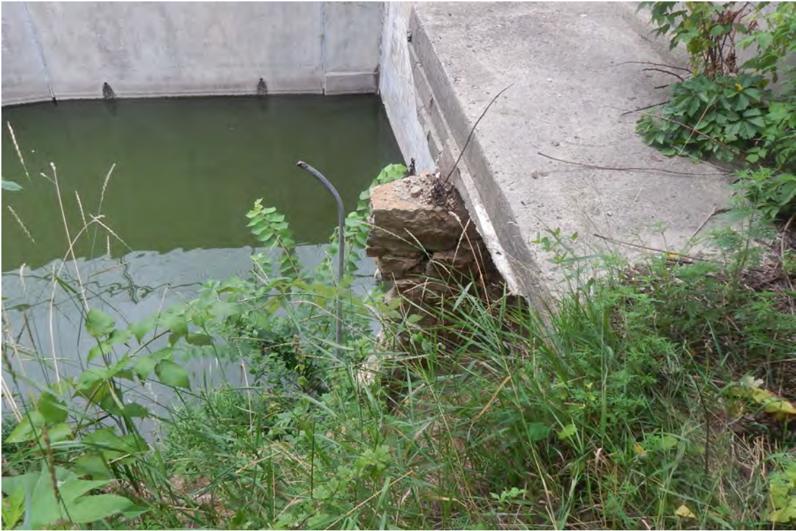
Photo 5 - Deteriorated Foundation/Retaining Wall
