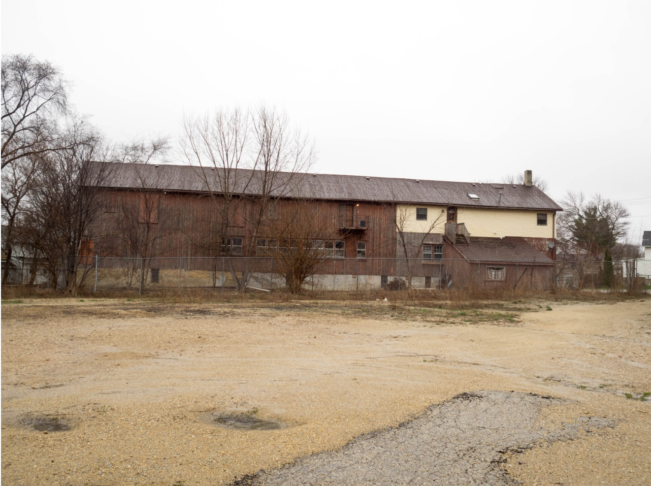
Former Carpet Warehouse building.
