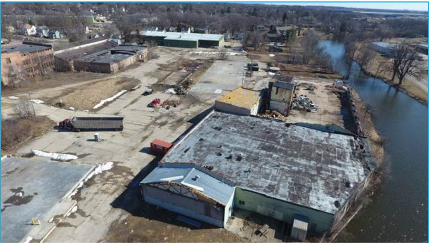
FIGURE 4: AERIAL VIEW OF THE HEART OF TID #8 SHOWING THE MILLFAB PROPERTY IN THE FOREGROUND AND THE HIGHWAY TRAILER BUILDING IN THE UPPER LEFT OF THE IMAGE.
