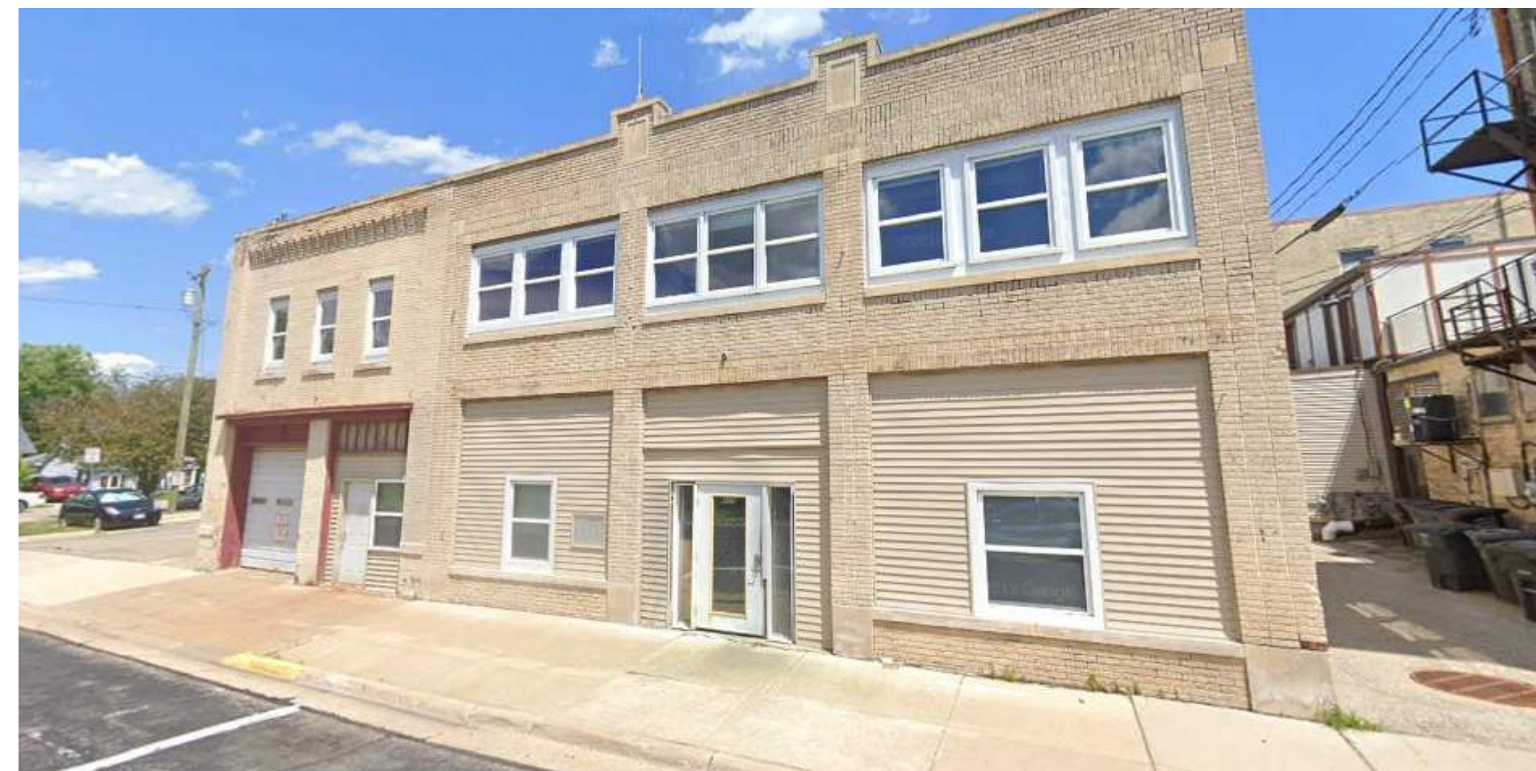
EXISTING STREET WATER ST FACADE
