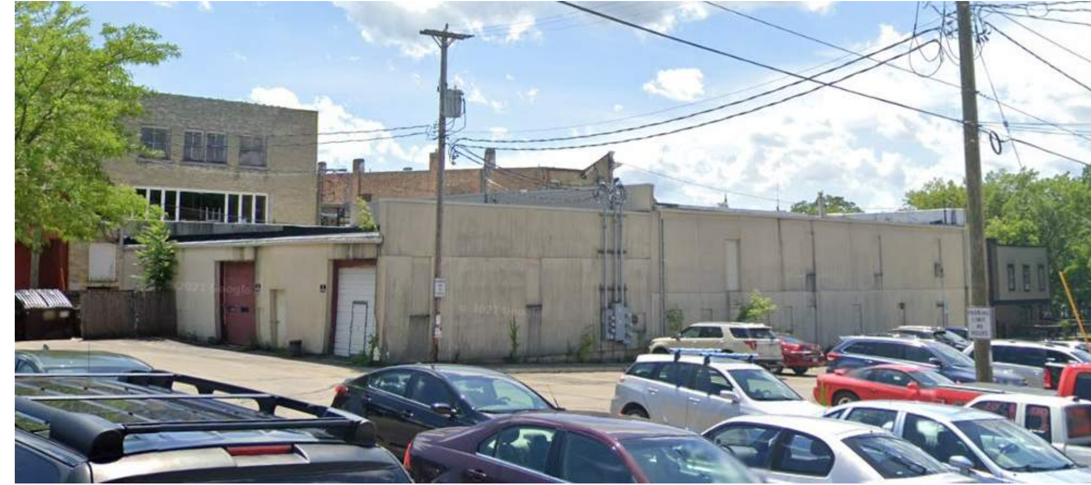
EXISTING NORTHEAST FACADE
