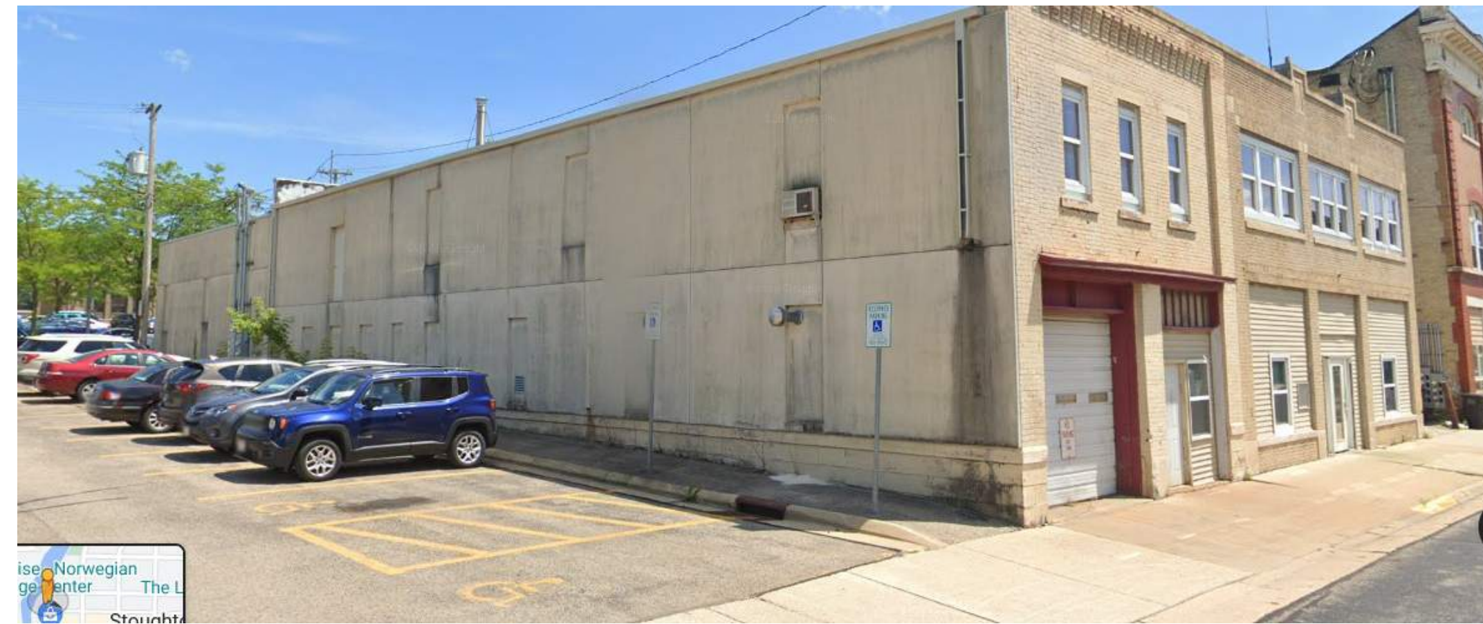
EXISTING NORTHWEST FACADE
