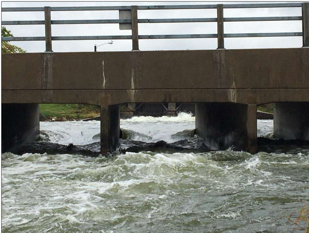
Figure 1. Existing box culverts under 4 th St. Date: October 22, 2019. Approximate discharge at Forton St gauge: 920 cfs.
